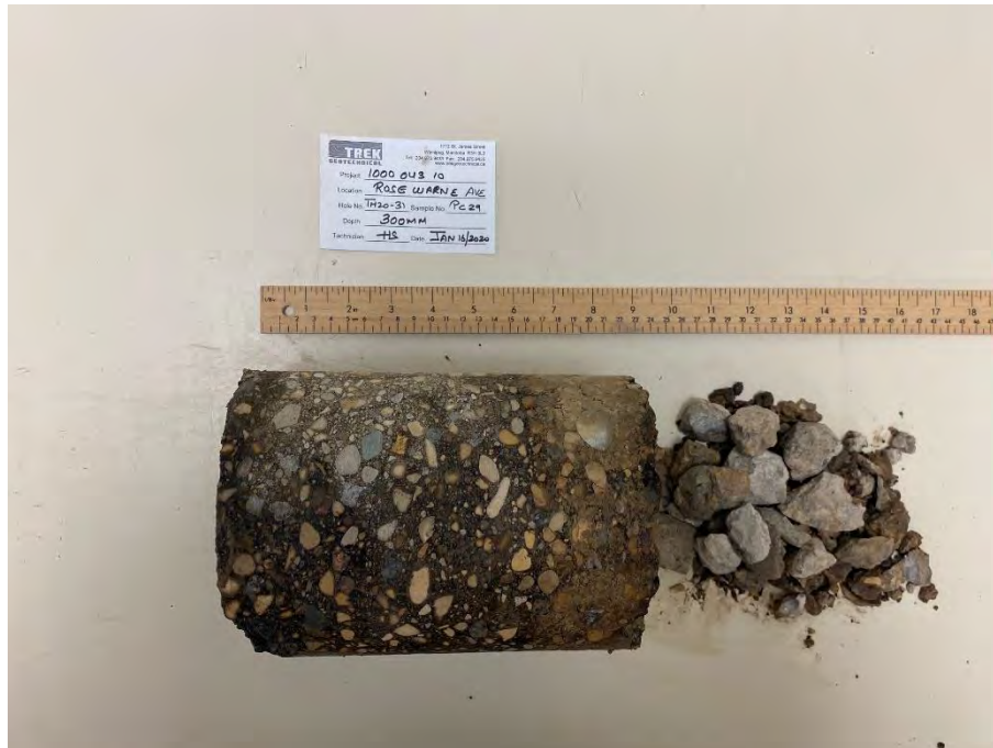
Photo 5: Pavement Core Sample at Test Hole TH20-31
