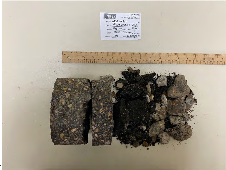
Photo 3: Pavement Core Sample at Test Hole TH20-29
