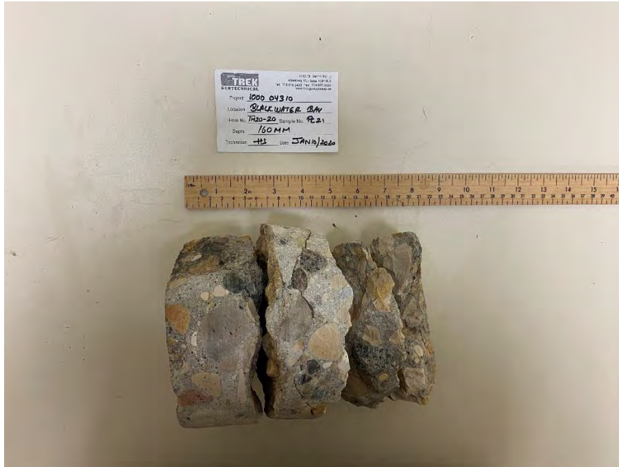
Photo 1: Pavement Core Sample at Test Hole TH20-01
