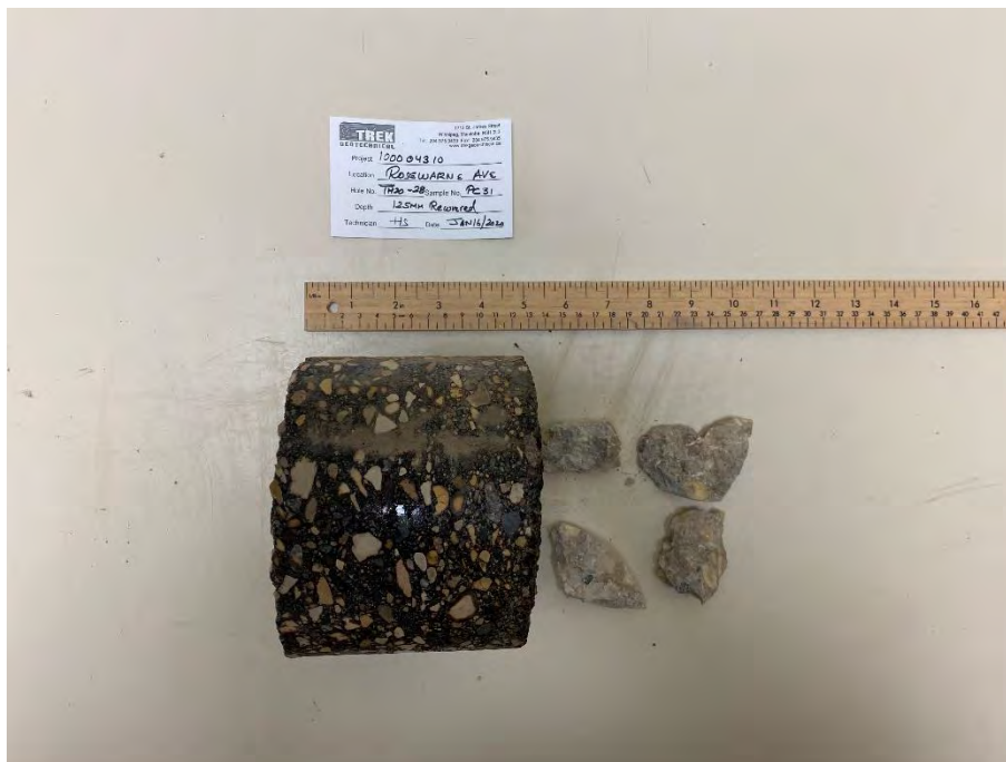
Photo 2: Pavement Core Sample at Test Hole TH20-28
