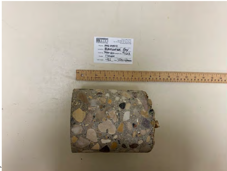
Photo 3: Pavement Core Sample at Test Hole TH20-03
