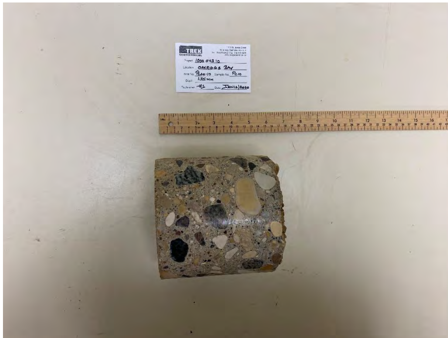
Photo 4: Pavement Core Sample at Test Hole PC20-10
