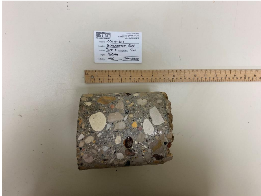
Photo 1: Pavement Core Sample at Test Hole PC20-01
