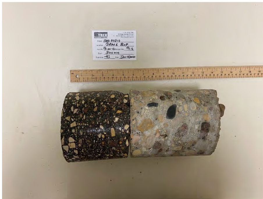
Photo 4: Pavement Core Sample at Test Hole PC20-16
